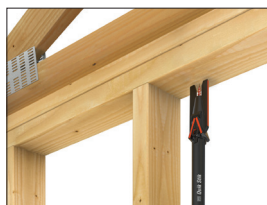
Gable end truss installation.
