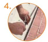
Pour concrete, let set and then pull tear-strip. Apply sealant per specifications.
