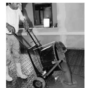
Using the pouring device
