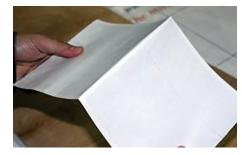
Create Vertical CREASE B. Fold FlexWrap™ in half, lengthwise, and create sharp crease at the fold.
