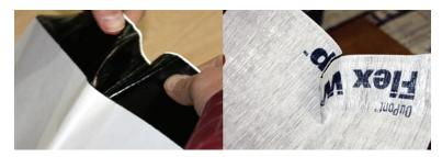
7. Form Recessed Window Corner. Remove narrow-width release paper and, using the creases made in Step 6, carefully press together the exposed butyl within the corner fold to create Recessed Window Corner. Repeat with the 3 remaining 12" pieces of DuPont™ FlexWrap™.
