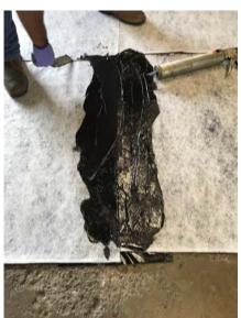
Place the DETAIL FABRIC into the POINTING MASTIC making sure that it is fully embedded and roll press into place.
