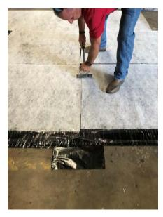
Apply a 12" (304.8 m) band of the POINTING MASTIC onto this overlap at a thickness of approximately 60 mils.
