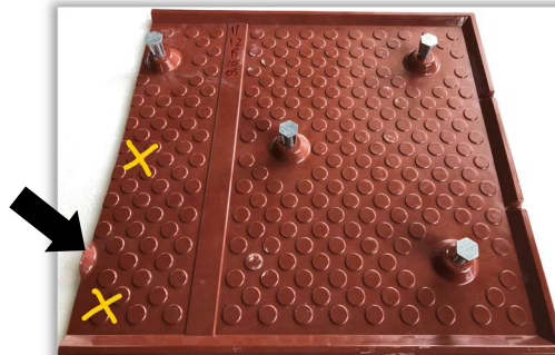
Figure 15: Underside of field cut CIP Replaceable panel. Note location of removed anchor (arrow) and locations of new supplemental anchors (yellow 'x') along 24-inch cut edge.
