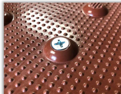
Figure 17: View of dome with new anchor fastener installed.
