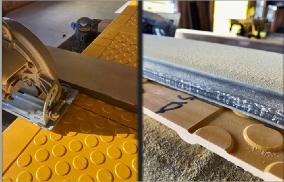
Figure 5: Cutting across bottom of Surface Applied tactile panel and closeup of cut edge
